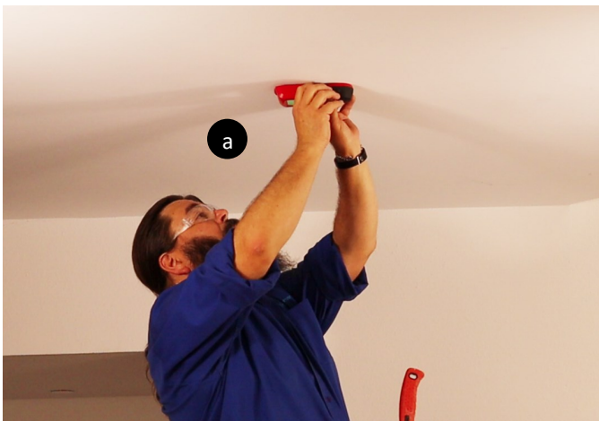
Choose desired location that is between ceiling joists
