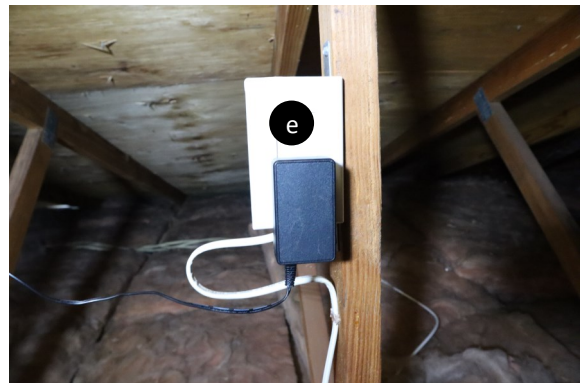
Plug power cord into outlet in attic. Run receiver end of cord to cut ceiling opening.
