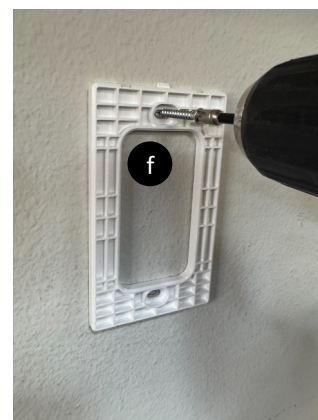
Place wall plate over wall anchors and fasten to wall
