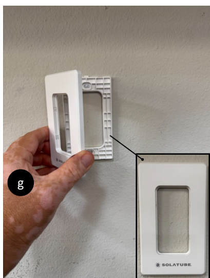
Place cover over wall plate and press to snap into place
